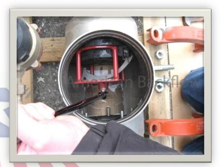
Place plate side of tool on studs of #2 check.
