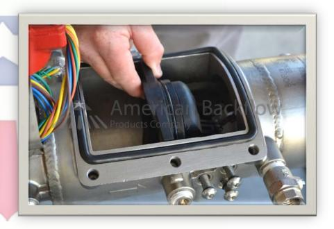
Do not tighten retaining screws until check 1 is installed.
