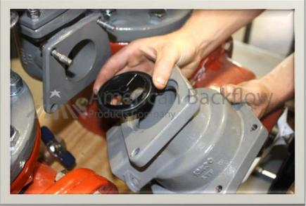
Place the module on a flat surface with lower guide facing up.
