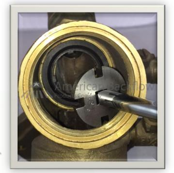
Place the tool on the correct size socket wrench.
